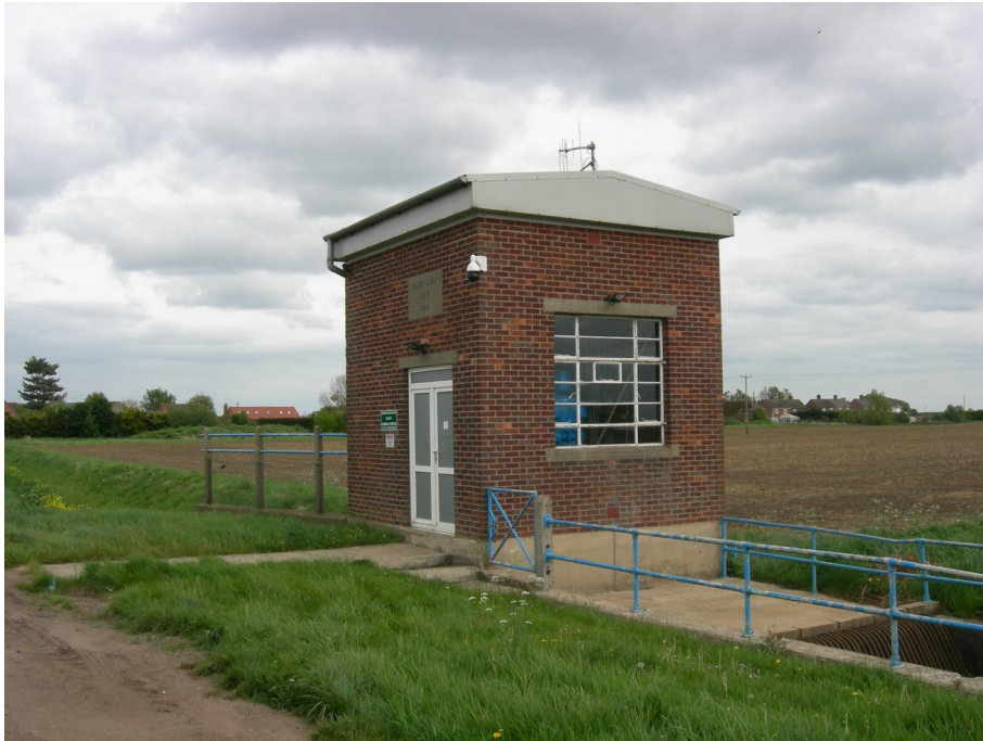
Above: Pumping Station on A151 Spalding Road
