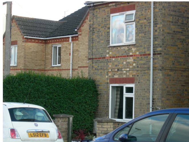
Above: Stanley Street - ribbon brickwork
