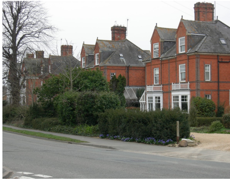
Above: Westbourne Villas on West Road
