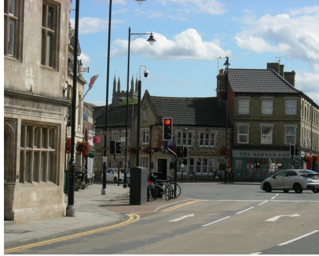
Above: View B. The tower of Abbey Church and Market Place from North Street
