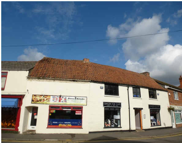
Above: Mansard roof on Abbey Road
