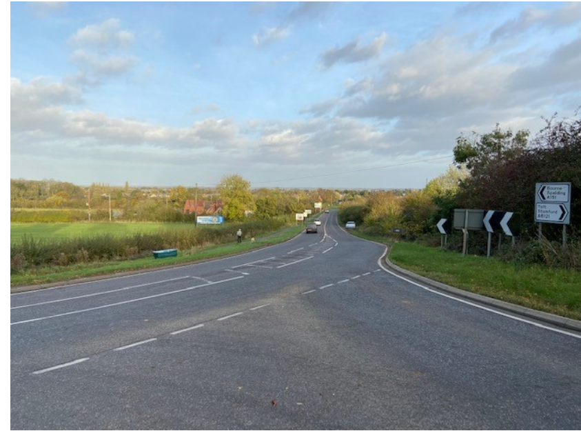
Above: Entry to Bourne from the west
