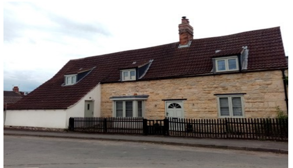
Above: Victoria Place. 18 th century stone former farmhouse with catslide and sloping dormers in local vernacular manner.
