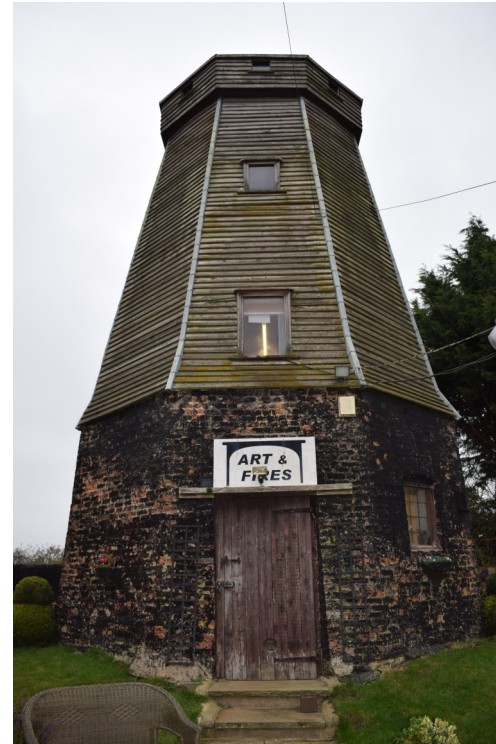
Left: Dyke windmill – original opened around 1650 to power the water pumps in Deeping Fen. Around 1840 it was dismantled and rebuilt in Dyke where it was used as a flour mill and to grind cattle food. It continued in use until 1926, the adjacent bakehouse producing bread for the village
