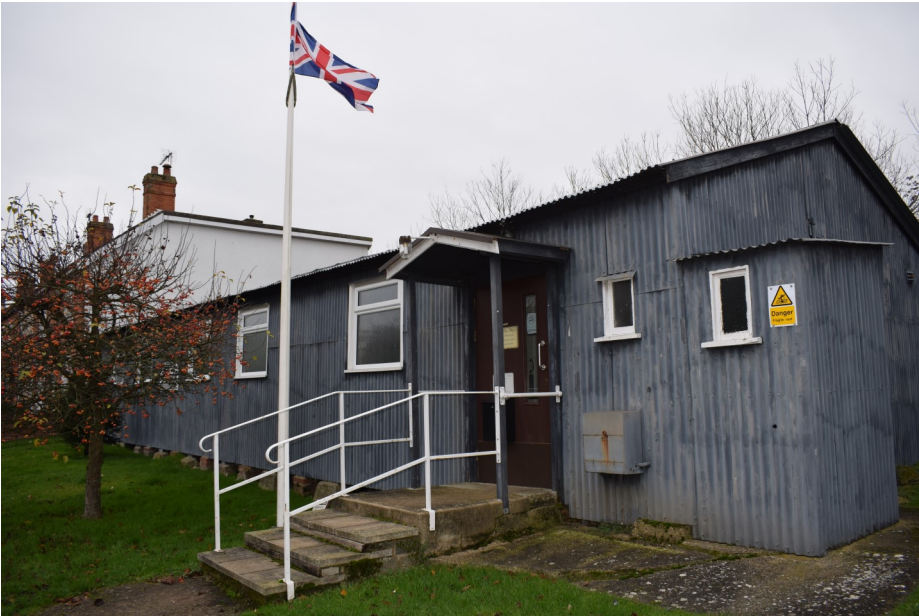
Above: The Village Hall—made of timber and cladded in corrugated iron, this started life as an army hut at Belton Park during World War 1
