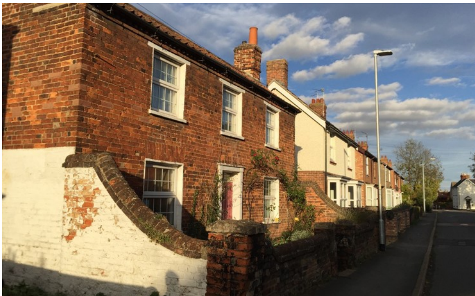
Above: good 18 th century double pile house with pantiled roof. Front range thought to be 1740, back 1760.
