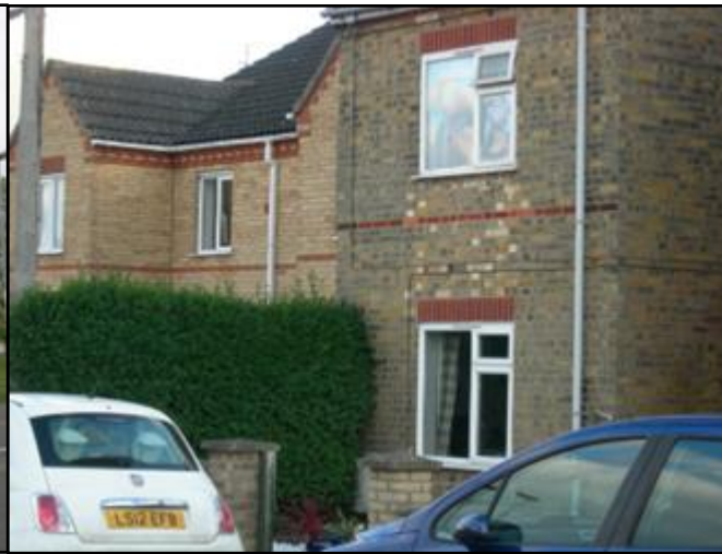
Stanley Street - ribbon brickwork
